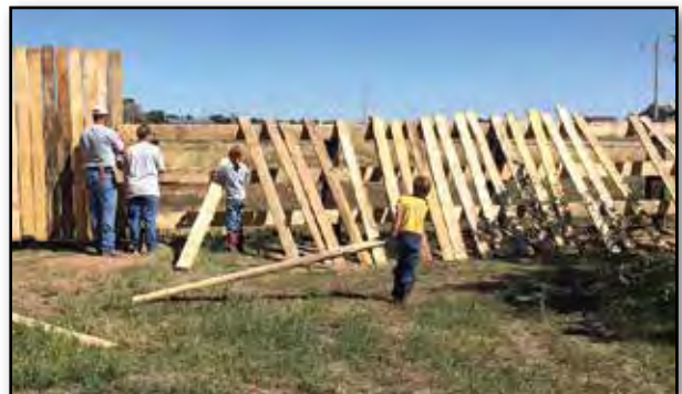
The crew building a windbreak around the new pens.
